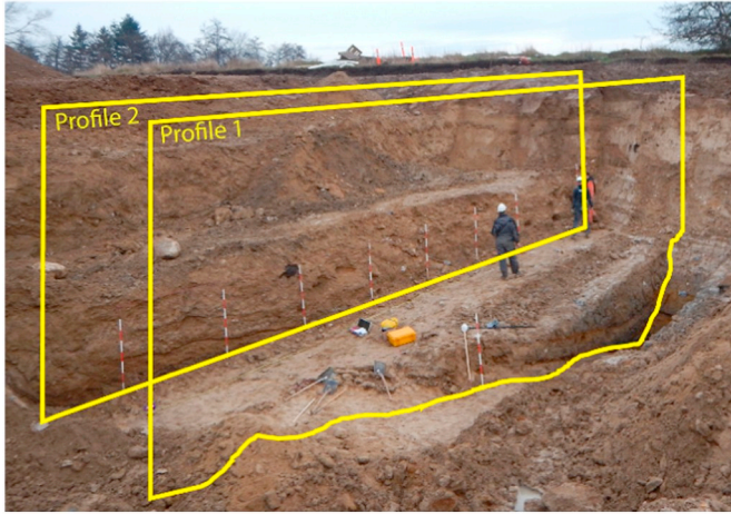
Fig. 5. Picture from the excavation with the geological profiles P1 and P2 superimposed.
